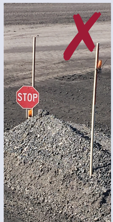
Sign required to be 1.5m above road surface. Flashing lights incorrectly mounted.
